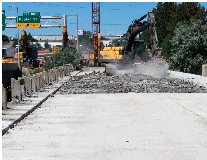
The F Street Bridge in Casper had to be demolished first so the contractor could begin demolition on the northbound I-25 bridge over the North Platte River.
