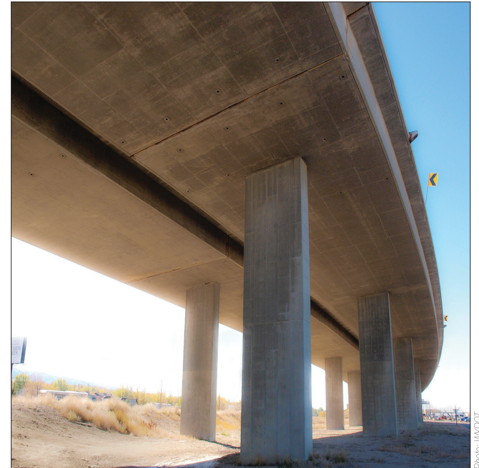
A look of the Walsh Drive bridges from below.
