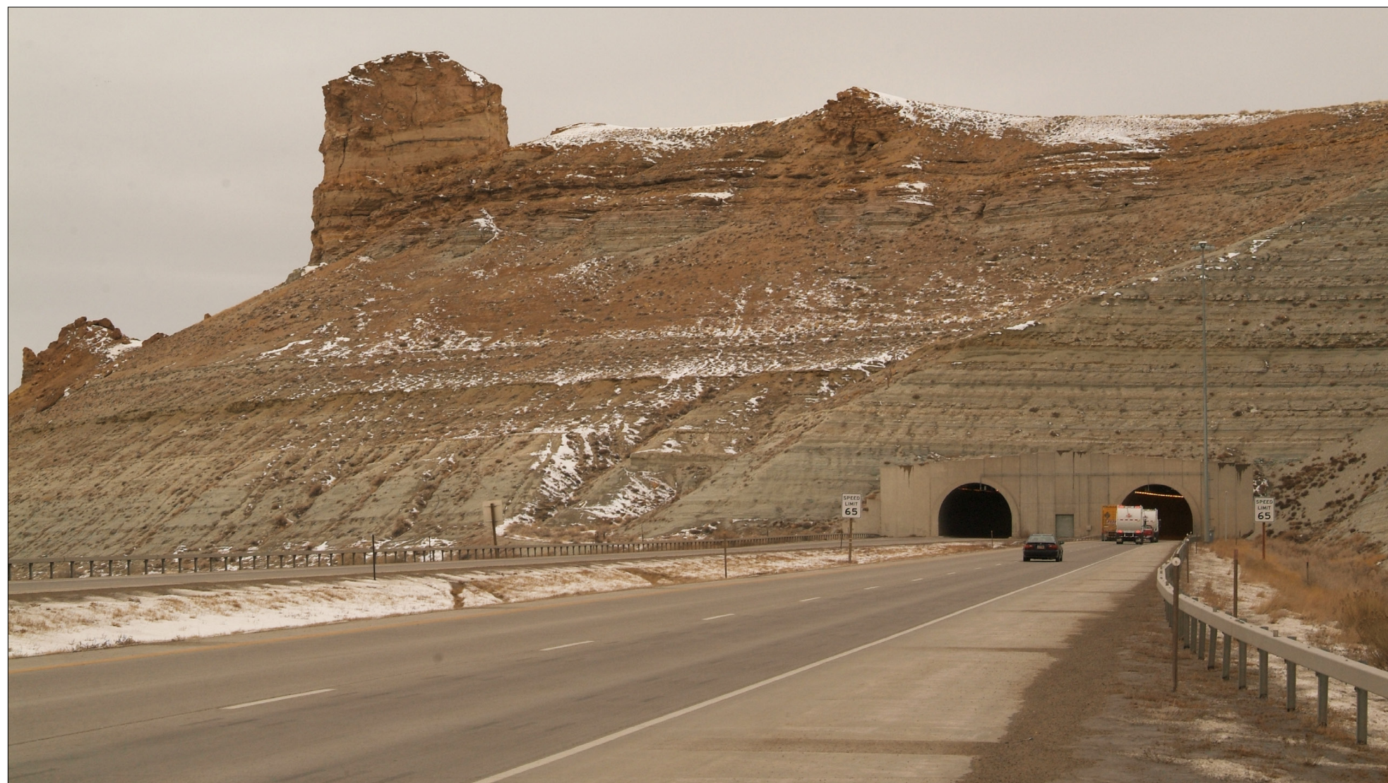
Green River Tunnel on I-80
