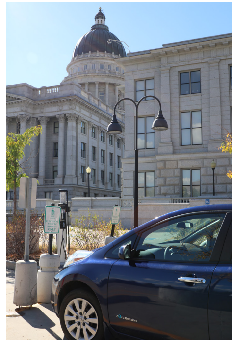
Figure 4: EV charging stations located at the Utah State Capitol in Salt Lake City, Utah.
