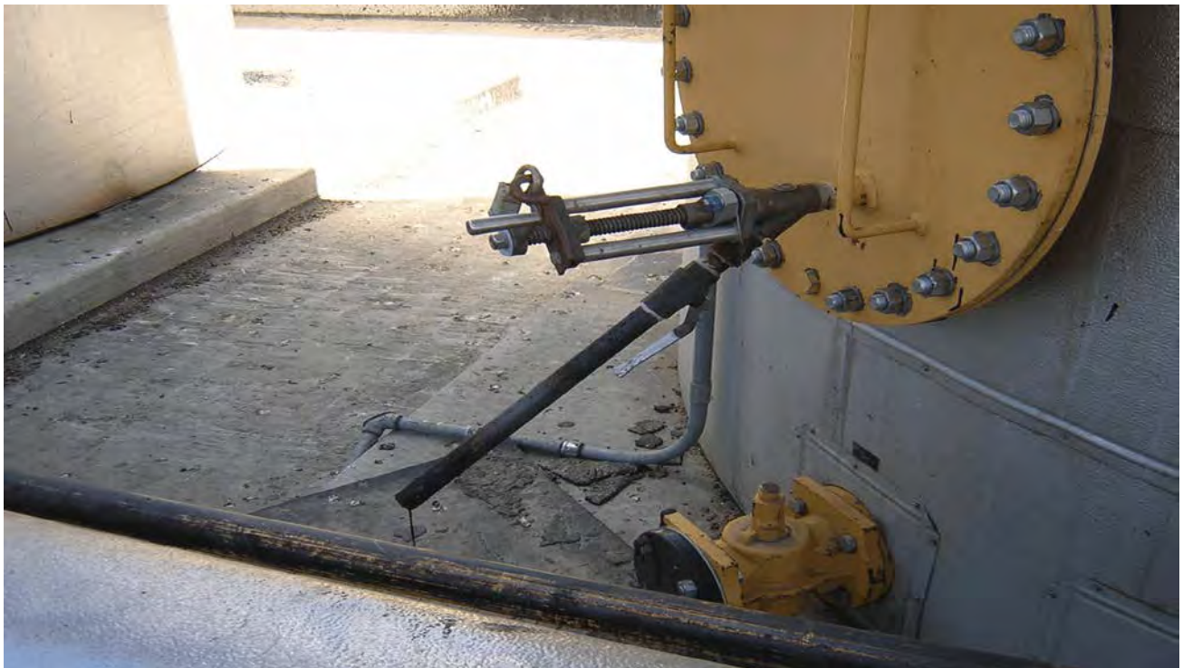
Figure 1 - Typical Sampling Valve for Tanker
