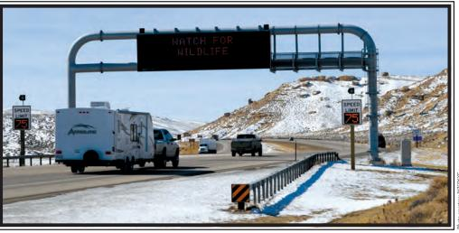
Accident rates have decreased by 50 percent on Interstate 80 between Rawlins and Laramie with the use of variable speed limit signs.
