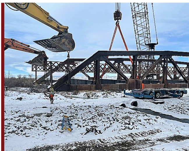
D5 CONSTRUCTION removing old steel truss bridge from Cottonwood Creek.
