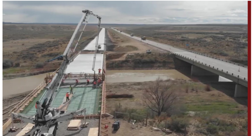
I-80 bridge over Black Fork's River west of Green River
