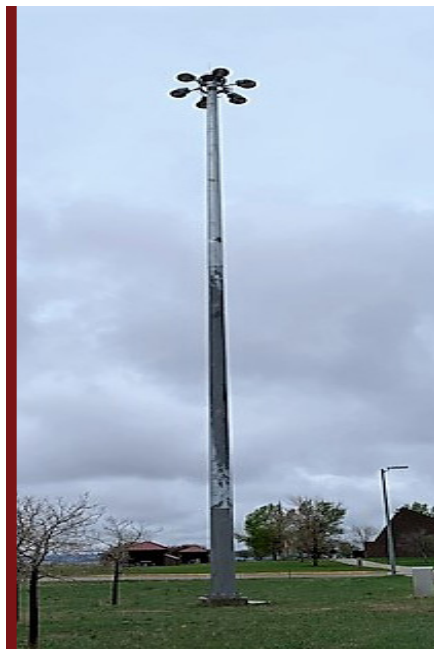
BRIDGE completed wind tunnel testing and design for the new high mast light towers. High mast light tower failure is a national issue, and WYDOT's valuable research resulted in important updates to national design standards.
