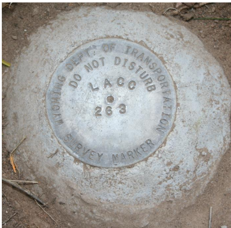
Figure IV-1. Project control monument.
