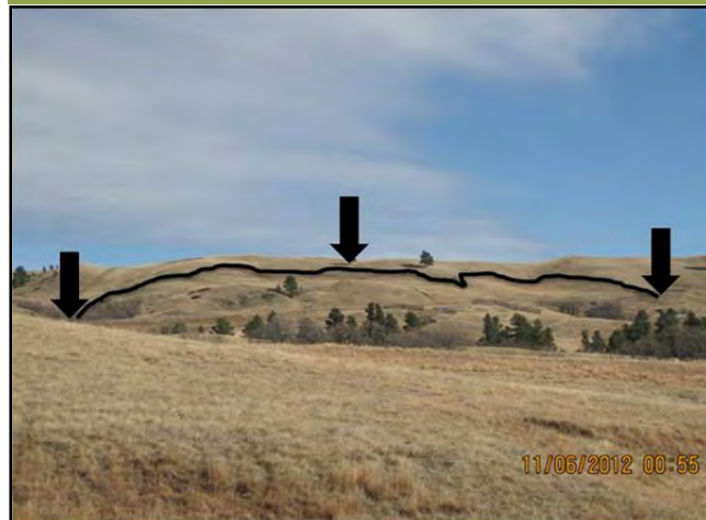
Figure 1-4. Extent of Rupe Hill landslide
